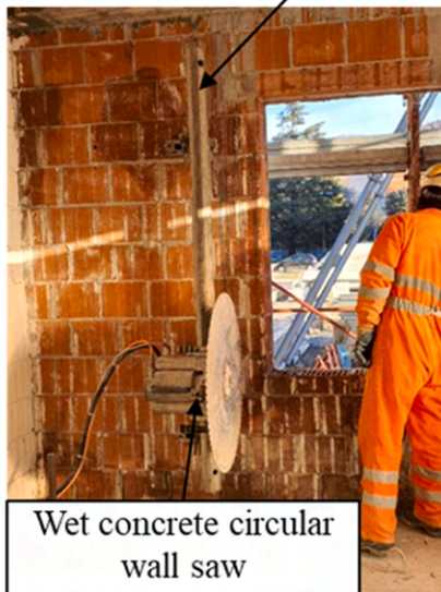
Fig. 2. Preparation of the one-way spanning walls (inside view).
