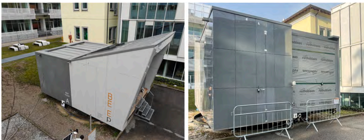
Fig. 3. View of the BEE Lab testbed after completion, in the context of the Lecco Campus of Politecnico di Milano.
