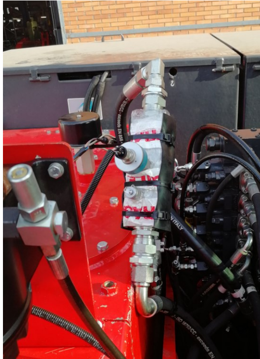
Figure 5.2 Hydrotechnik QT-400 flow sensor installation on the M15e.
