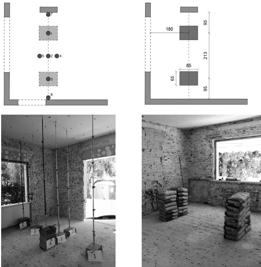
a) Level below the one to be tested
