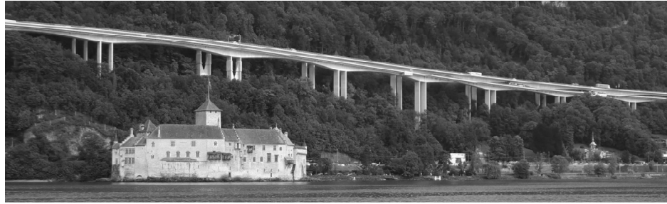
Figure 2.2-12: Chillon viaducts along Lake Geneva [Brühwiler et al. , 2015].
