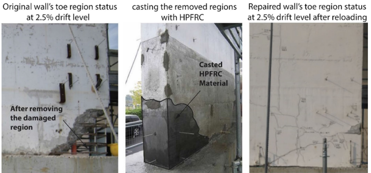
Fig. 2 The repair intervention of the tested wall and the obtained results. Modified from Preti, Meda [14]
