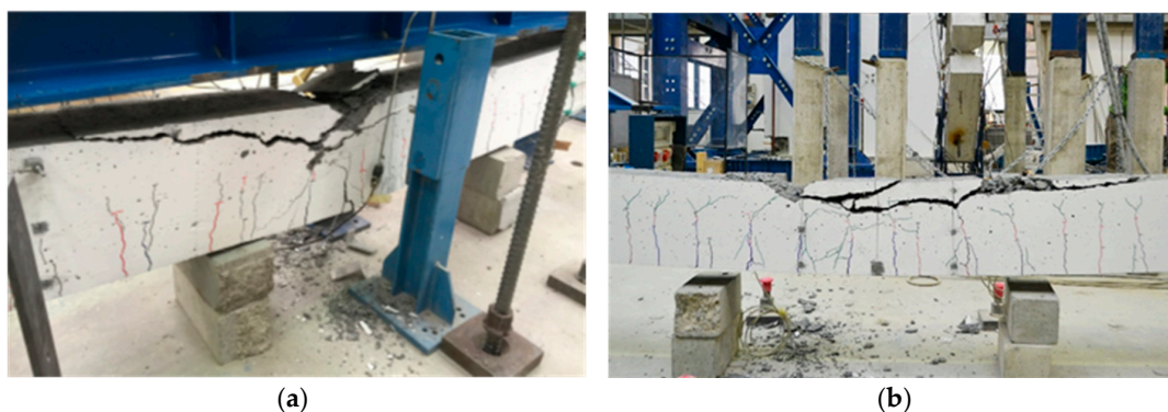
Figure 11. Concrete crushing, with yielding of rebar, for: AAC1-HC (a); and AAC2-HC (b).
