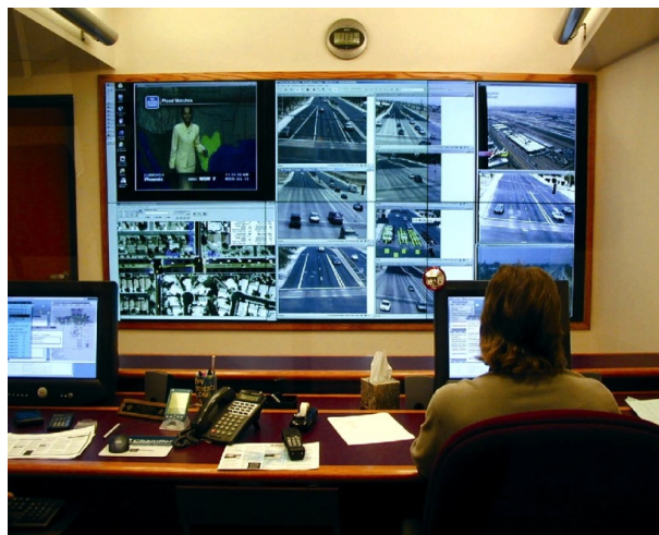
Figure 3 - Traffic management center, Arizona, US [3].
