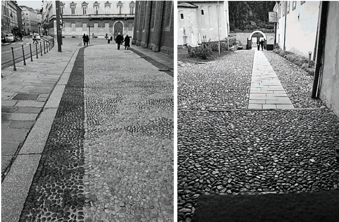
Figure 2. Refurbishment of historic cobble paving in Milano (left) and Merano (right)
