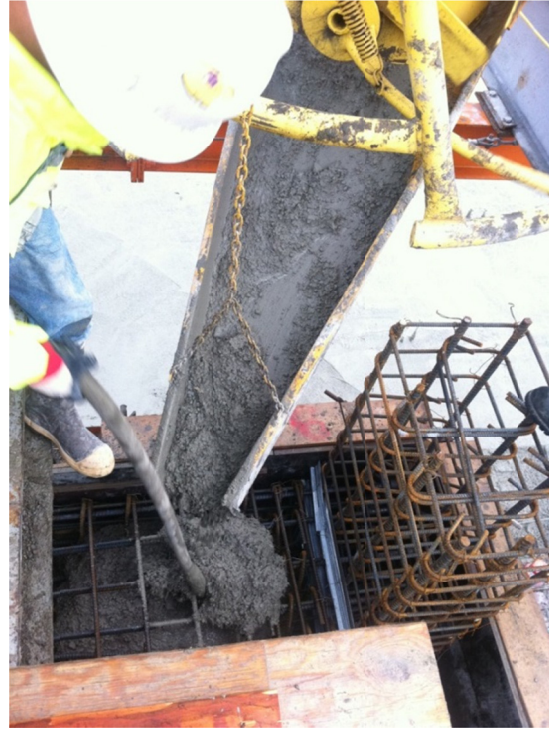
Figure 5. Casting of HPFRC in coupling beams
