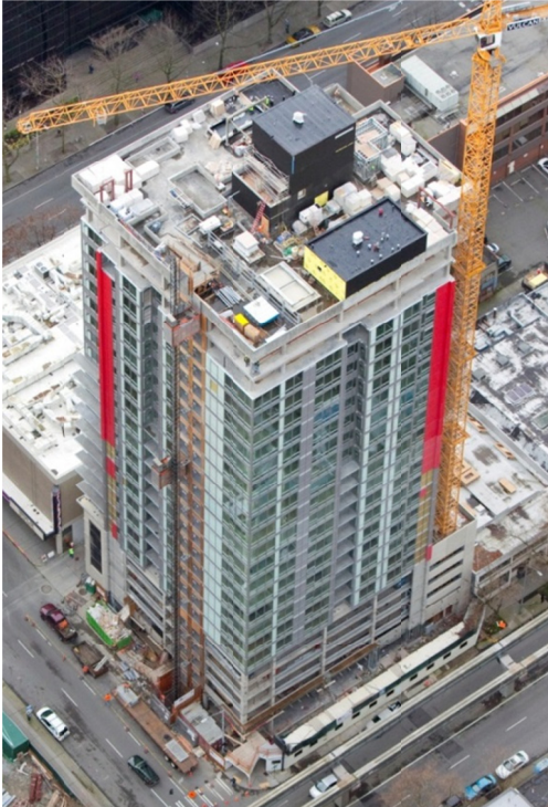
Figure 4. The Martin building, Seattle, WA
