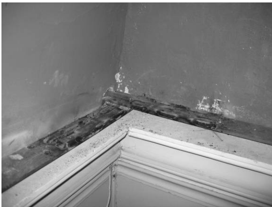
Figure 11. Detail of the internal perimeter ties hidden over the nave moldings in San Pietro Church, Roè Volciano, Italy.
