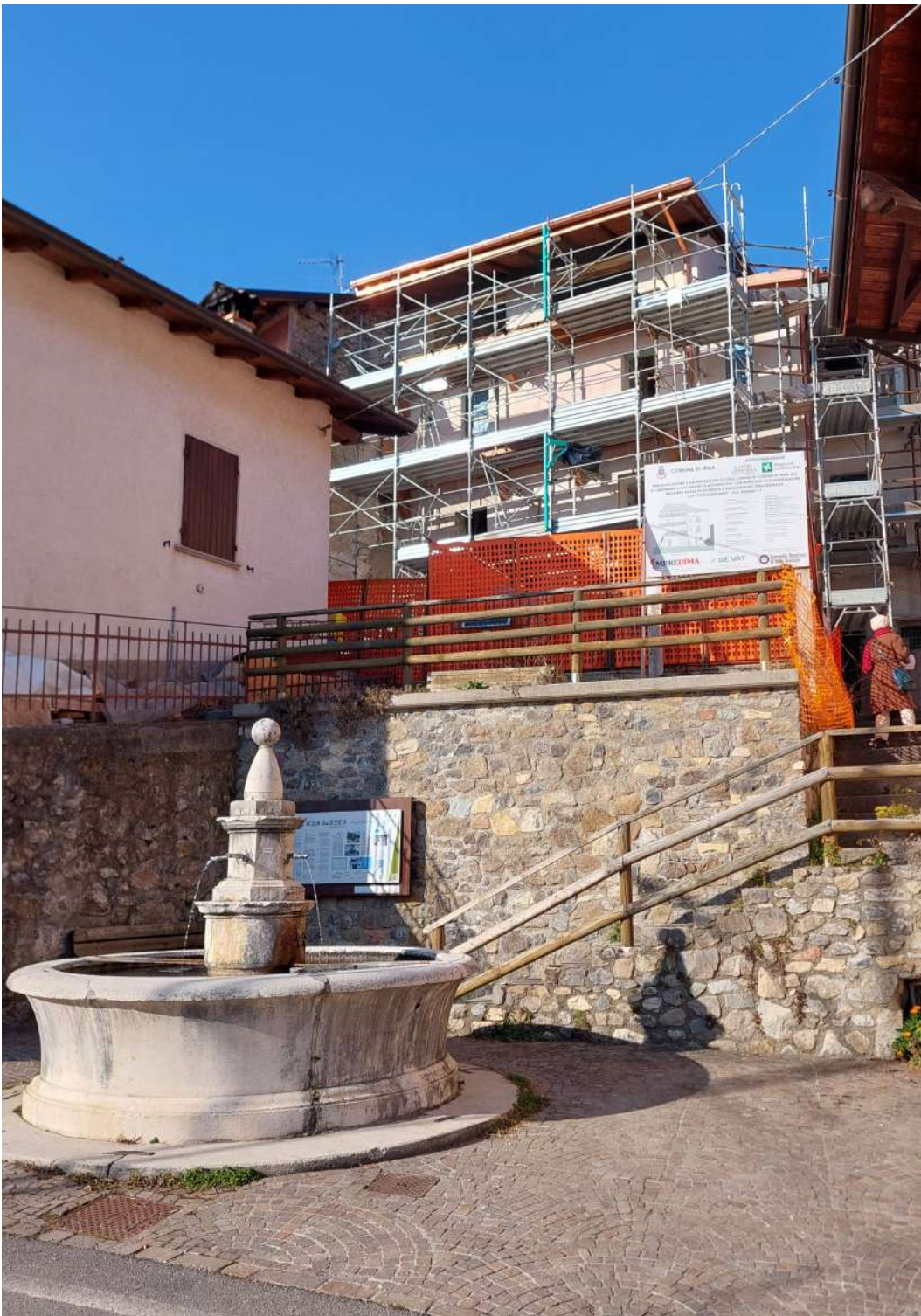
Figure 3. Casa Corsini near the fountain during conservation and restoration works, Irma, Italy, January 2026 (photograph by the authors)
