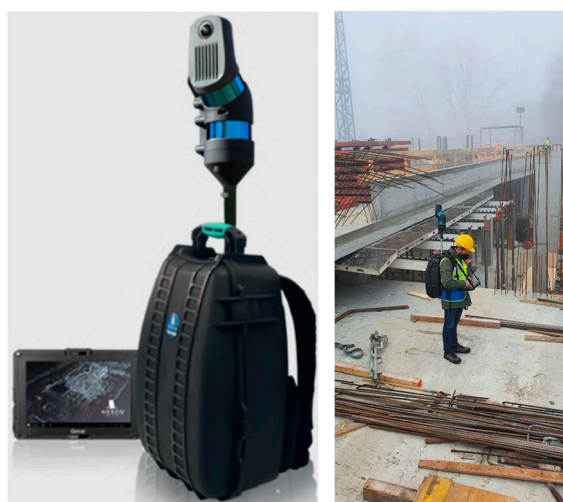
Figure 1. The wearable mobile mapping device (left) and its use during the monitoring phase at the construction site (right).
