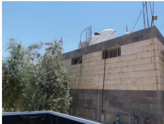
Figure G. 18 Elevated irrigation tank
