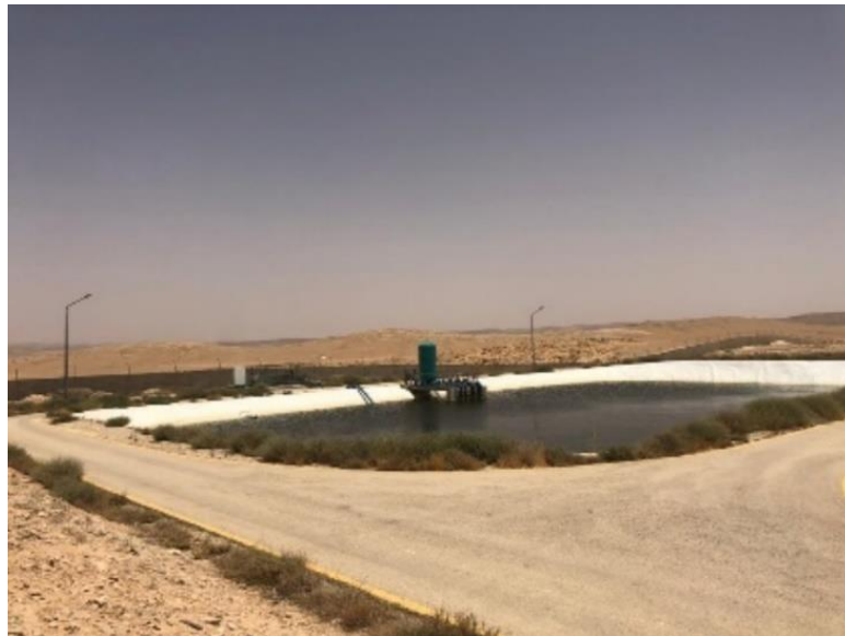
Figure A. 10 Final storage pond – Lajoun WWTP
