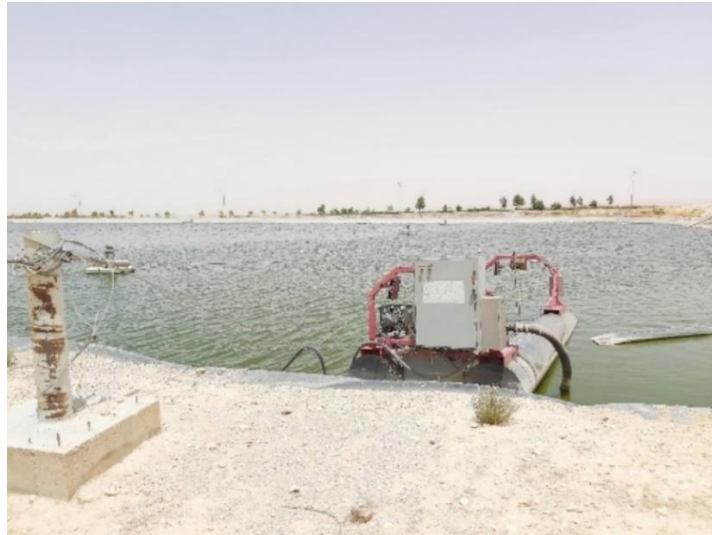
Figure A. 4 Sludge harvesting boat - Lajoun WWTP
