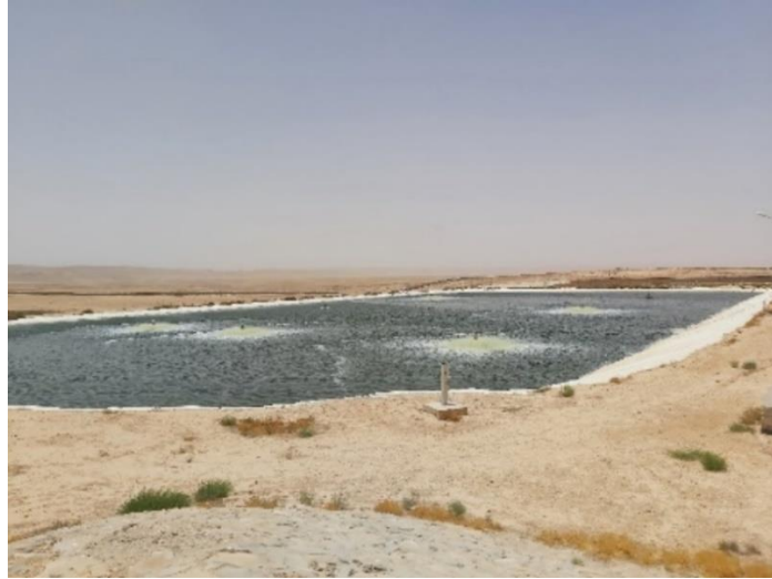
Figure A. 3 Aerated facultative pond - Lajoun WWTP
