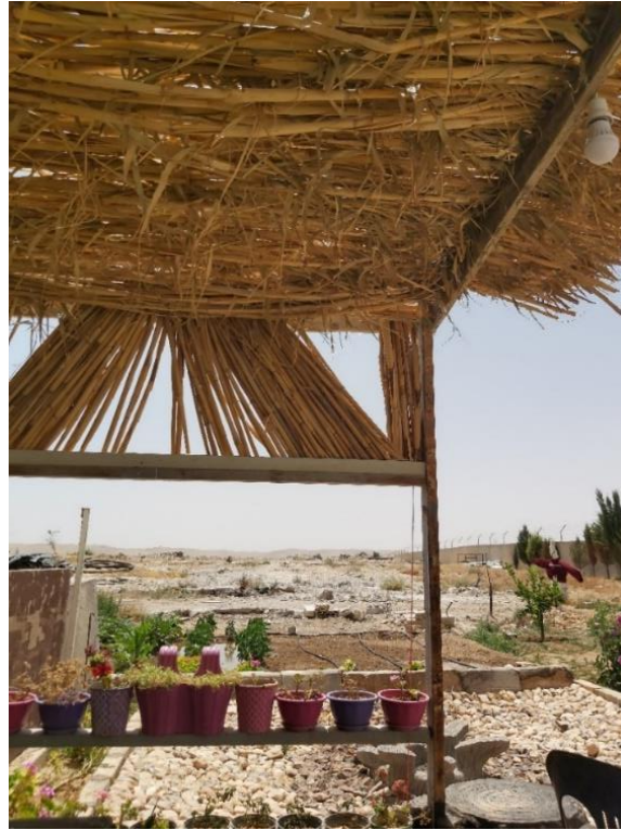
Figure A. 9 Reuse harvested reeds – Lajoun WWTP
