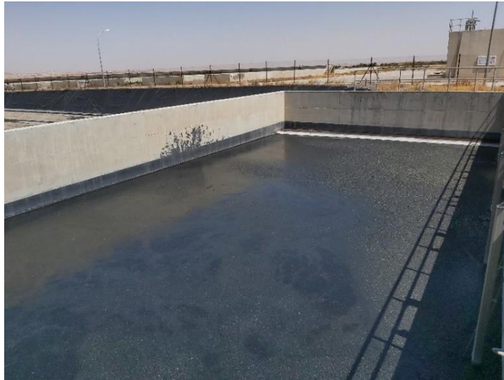
Figure A. 13 Denitrification Pond – Mafraq WWTP
