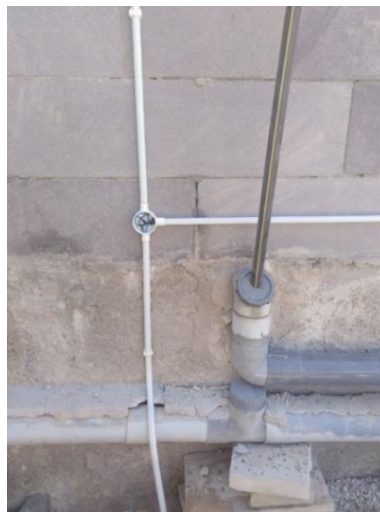
Figure G. 5 Recirculation to primary tank
