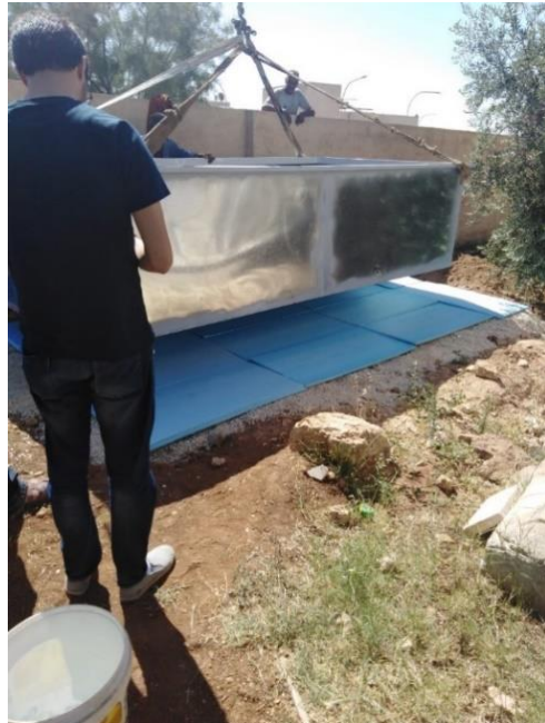
Figure G. 7 Installation of HFCW bed
