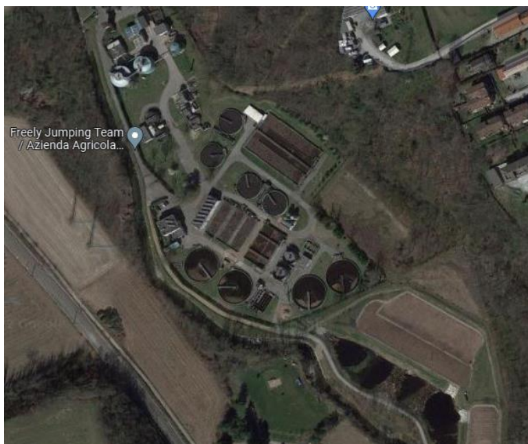
Figure 3. 36 Satellite image of Carimate WWTP 45°41'22.8"N 9°07'17.6"E
