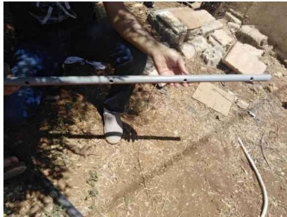
Figure G. 9 Even distribution – inflow pipe
