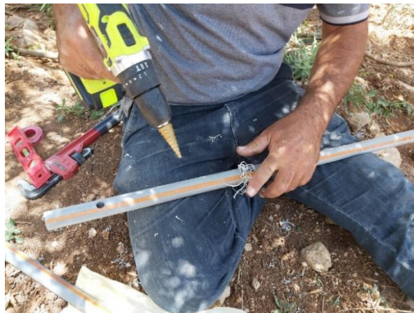
Figure G. 10 Even distribution – outflow pipe (2)
