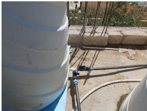
Figure G. 19 TGW disposal and reus connections
