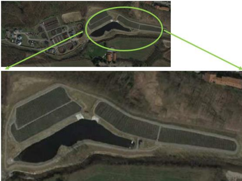
Figure 3.37 CWs in Carimat WWTP
