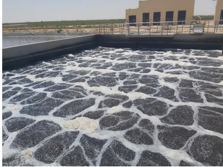
Figure A. 16 Nitrification Pond – Mafraq WWTP
