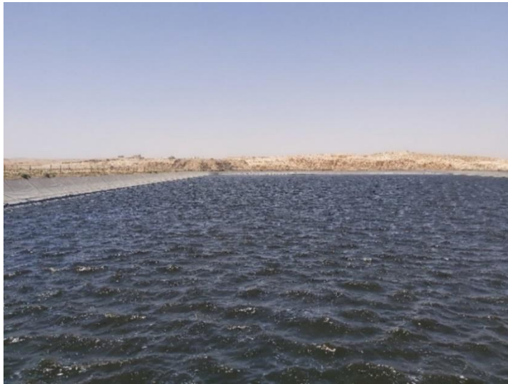
Figure A. 20 Treated wastewater storage pond – Mafraq WWTW
