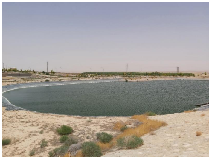
Figure A. 5 Maturation pond - Lajoun WWTP
