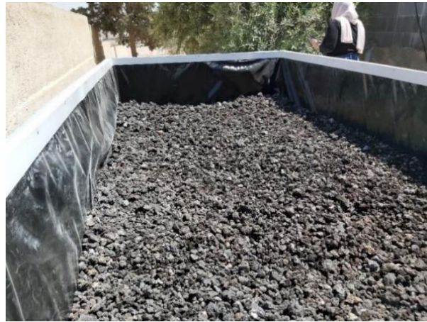
Figure G. 12 Distribution filter materials
