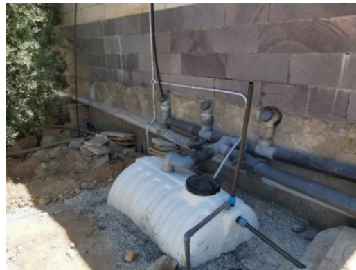
Figure G. 4 Primary settling tank – complete plumbing works
