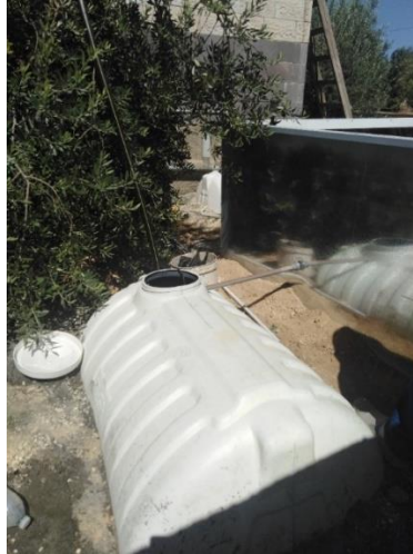
Figure G. 17 TGW Collection tank
