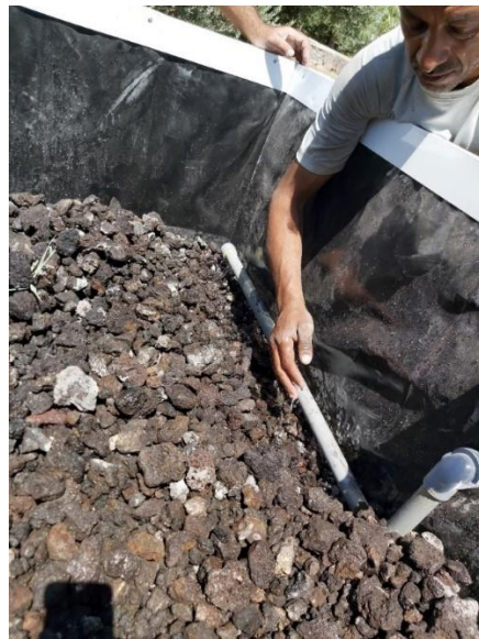
Figure G. 13 Flow testing
