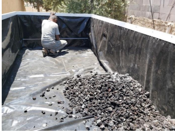
Figure G. 11 Outflow pipe installation
