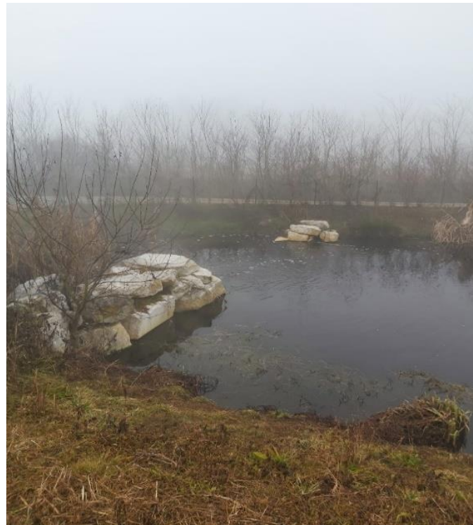
Figure A. 30 FWS CWs during winter season - Carimate WWTP
