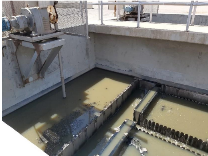
Figure A. 11 Grit removal – Mafraq WWTP
