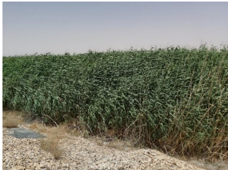
Figure A. 7 CWs - Lajoun WWTP
