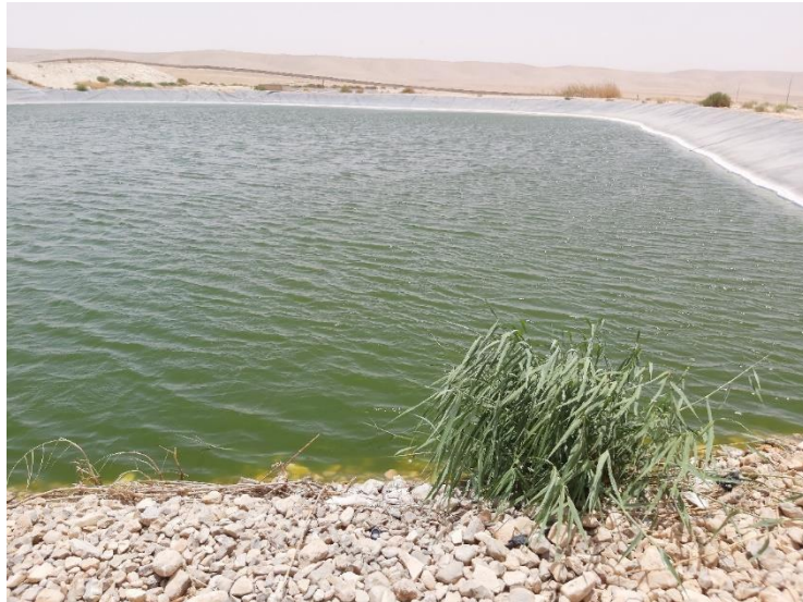
Figure A. 6 Rock filter - Lajoun WWTP
