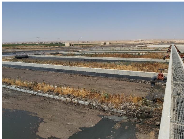
Figure A. 14 Sludge drying beds – Mafraq WWTP
