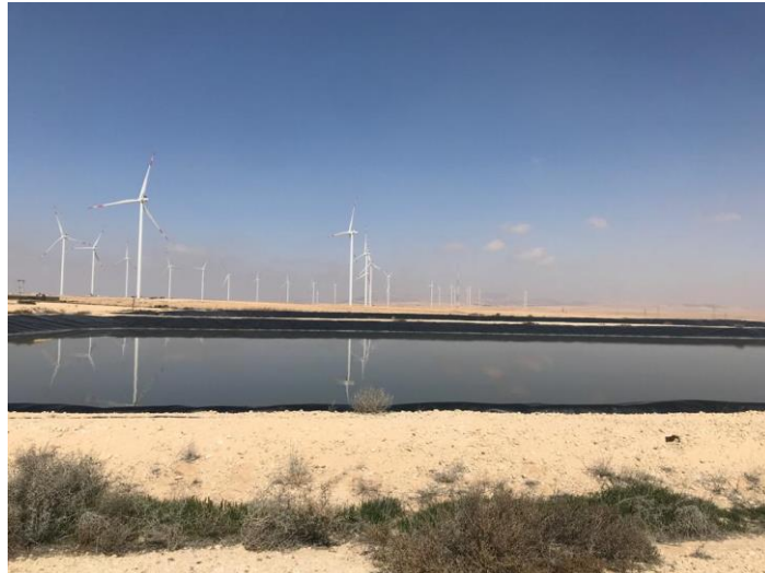
Figure A. 25 Evaporation Pond – Shoubak WWTP
