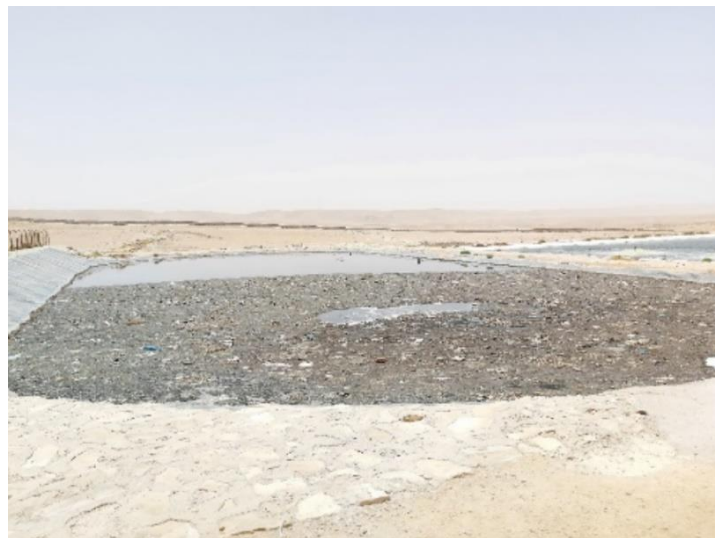
Figure A. 2 Anaerobic Pond - Lajoun WWTP
