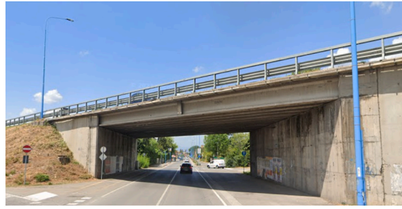
Fig. 2. The case study bridge.
