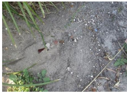
Sediment accumulation – build-up of fine sediments reduces infiltration and treatment.
