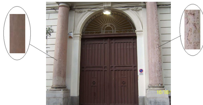
Figure 8. Palazzo Jung (Palermo). Altered column (on the right) and intact column (on the left).
