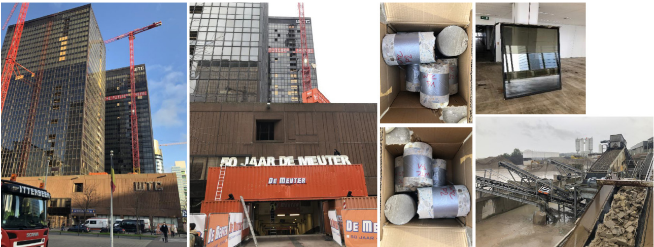
FIGURE 3: Local closed-loop recycling of concrete in the ZIN Project in Brussels, BE (Source: M. De Moradiellos, Drees and Sommer, ECESP Circular Talk 2021).
