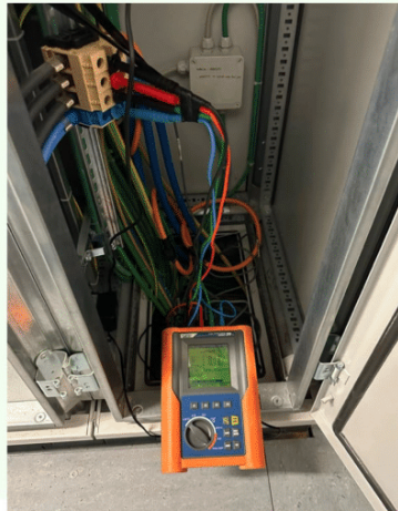
Power quality analyser and the energy consumption profile of an MRI working day
