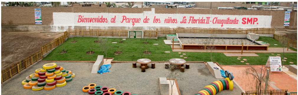
> Productive & Wastewater treatment Park "Children's Park", La Florida II, Chuquitanta © ILPÖ, University of Stuttgart
