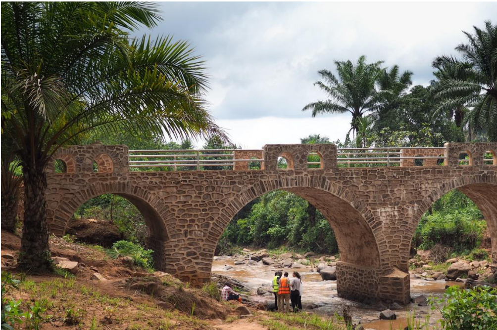
> Nyabigufa Bridge After Completion © Enabel Tanzania
