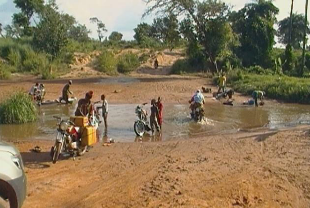
> Mazakuka - Construction of 3m x 2m Six Cells Box Culvert (before)
