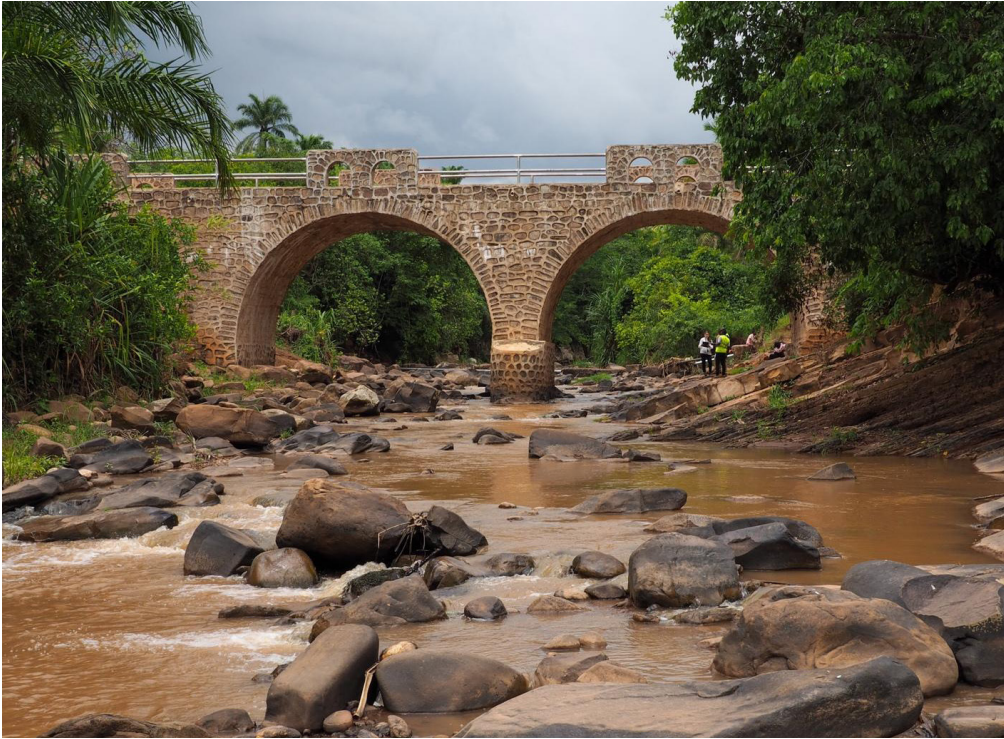
> Nyabigufa Bridge After Completion © Enabel Tanzania
