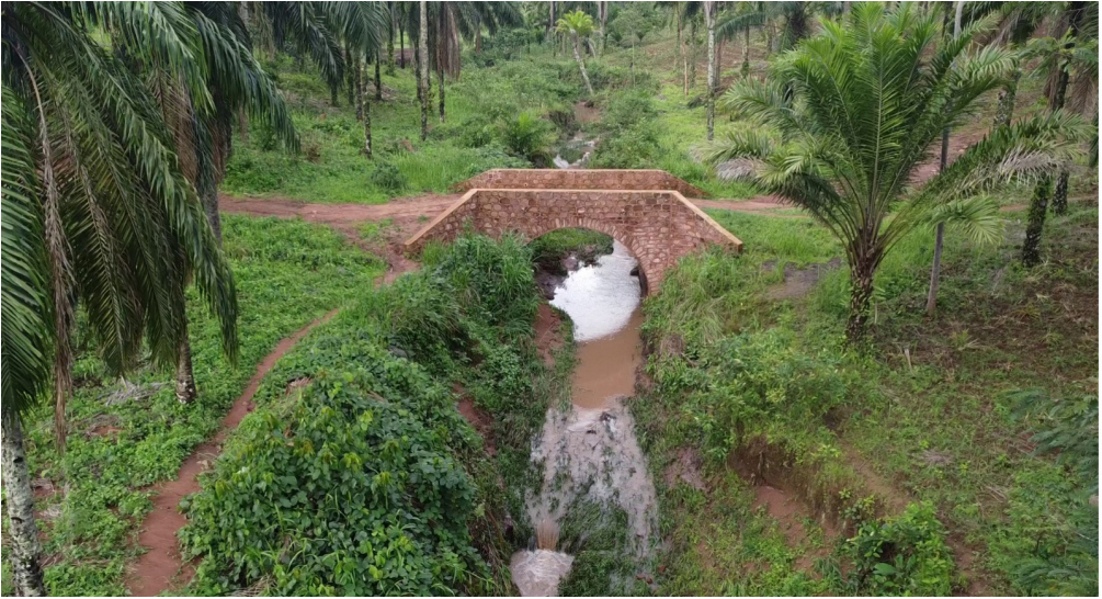
> Kilema bridge (6m span, 10 000 EUR) © Enabel Tanzania
