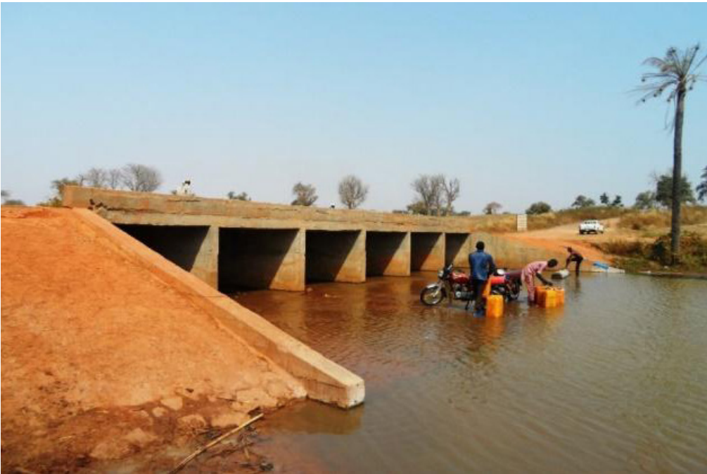
> Mazakuka - Construction of 3m x 2m Six Cells Box Culvert (after)
