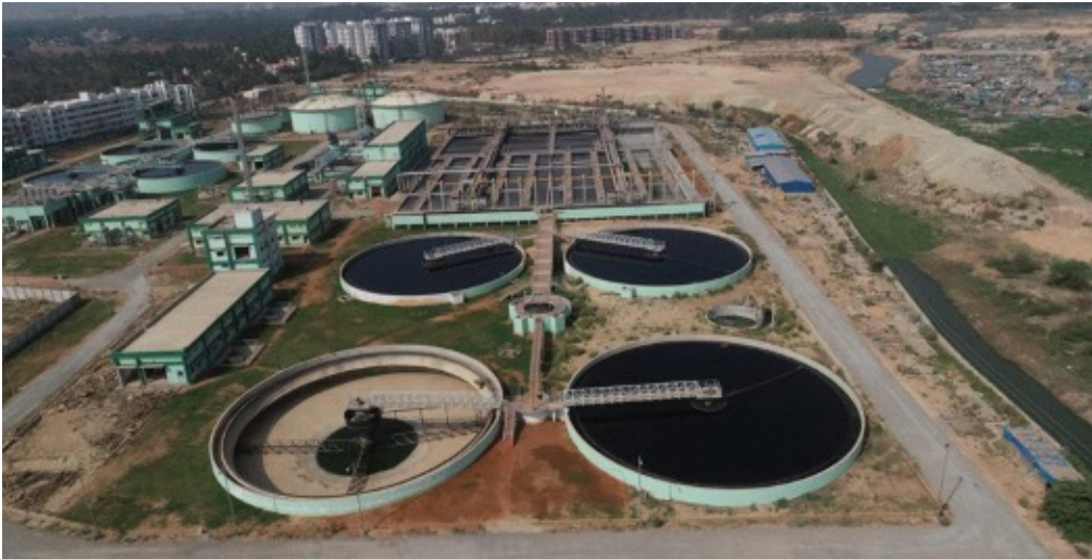
> Sewage treatment plant in bellandur, Bengaluru
