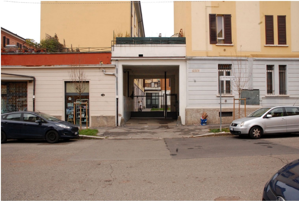
FIGURE 5 Gate installed at the entrance to one of the renovated courtyards in Congrega Apostolica's residential buildings in Porta Milano (photo by Marco Alioni, July 2025)
