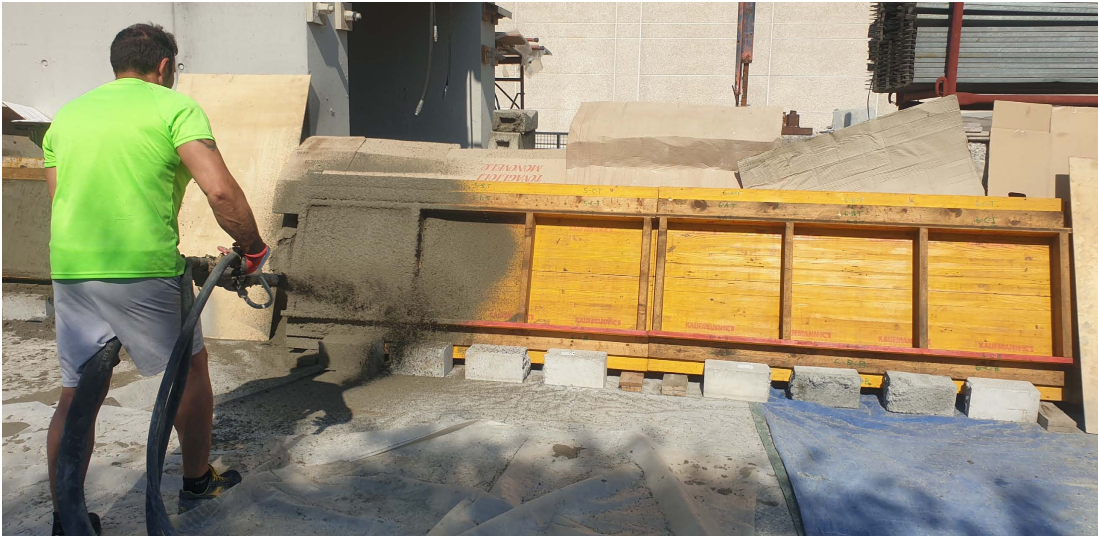
Figure 4.5: Outdoor spraying of the panels using the wet mix spraying process.
