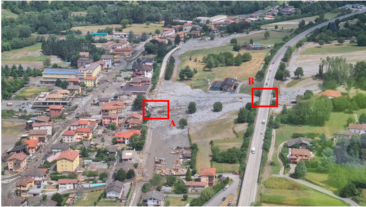
Figure 2.21 Helicopter view of Niardo the day after the debris flow event. From the image it is possible to assess the critical points in which the Re stream overflowed, which are located in correspondence of the railway bridge (downstream, A) and the highway bridge (upstream, B).
