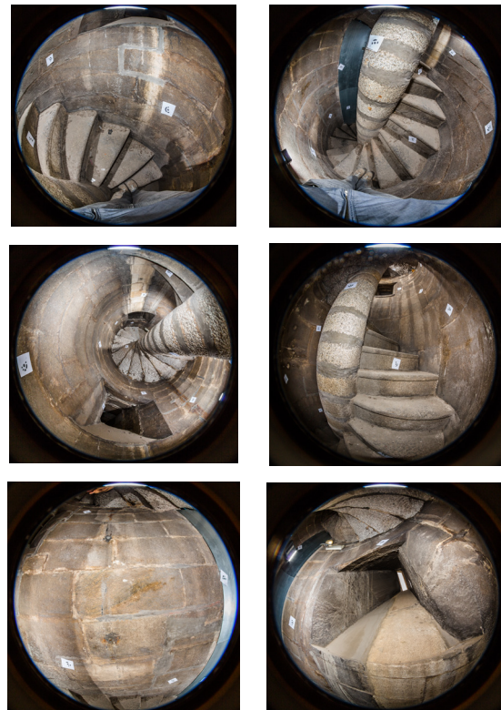
Figure 10. Five pictures which compose the capturing geometry, plus one detail picture (bottom right) of one opening.
