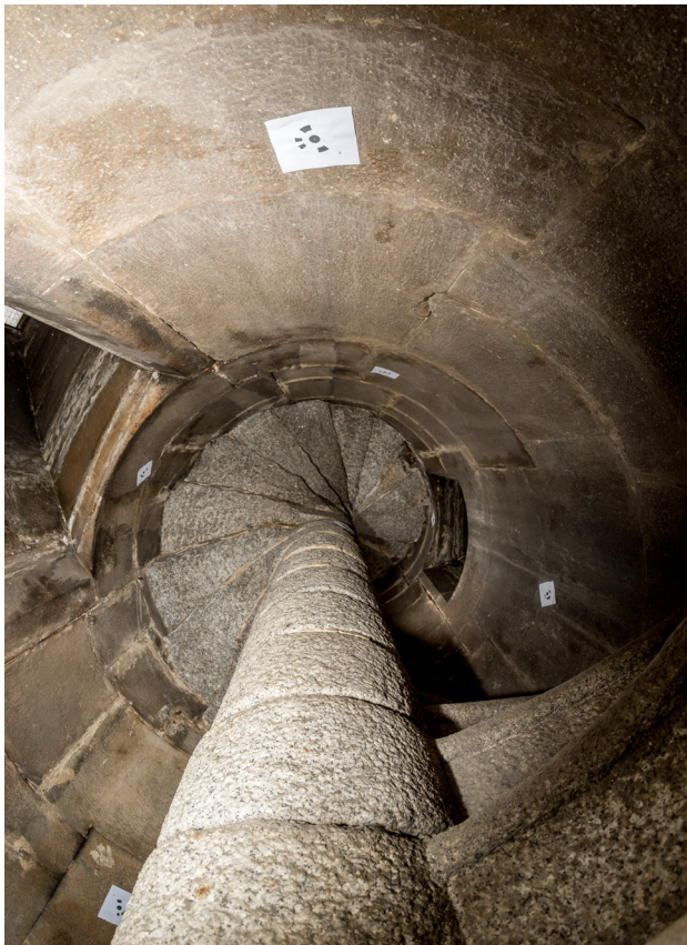
Figure 9. Internal view of the Minguzzi staircase during the photogrammetric survey.
