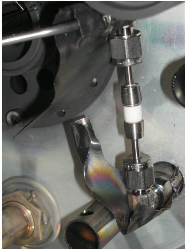
Figure 7.22: Gas connection protected by Tantalum sheet
