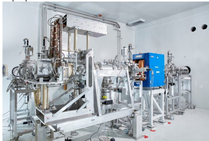
Figure 1.6 The Front-End bunker in an advanced installation phase.
