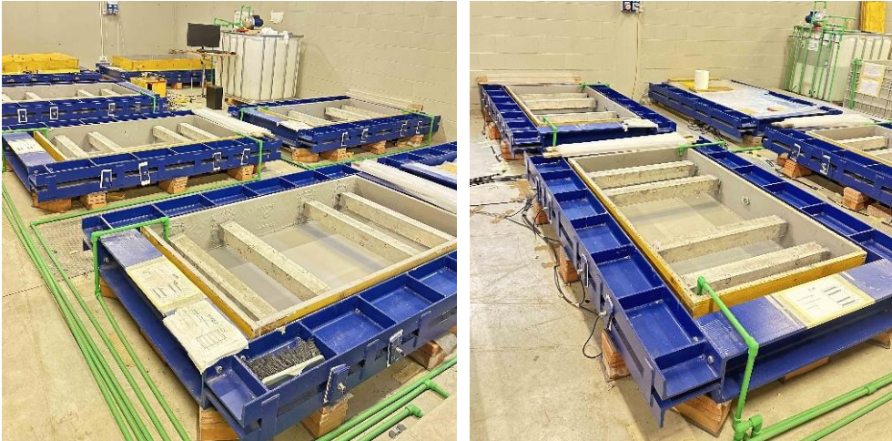
Figure 3.5-3. Tension ties placed in the water storage tank after applying waterproof paint.
