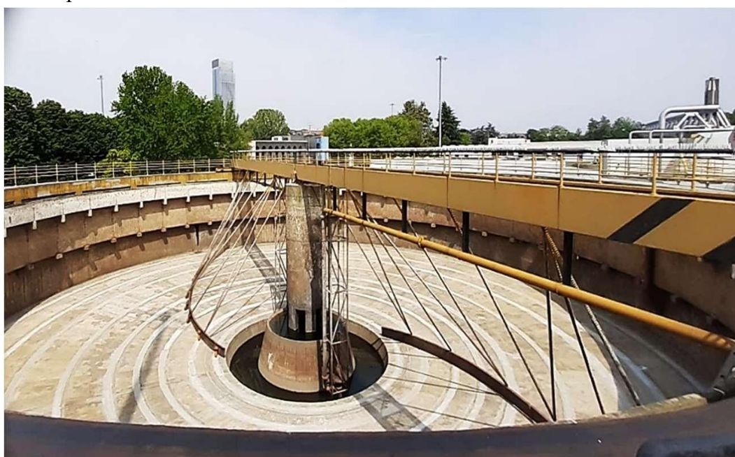
Figure 4. 17 Horizontal static pre-decanter – Source SMAT S.p.A
