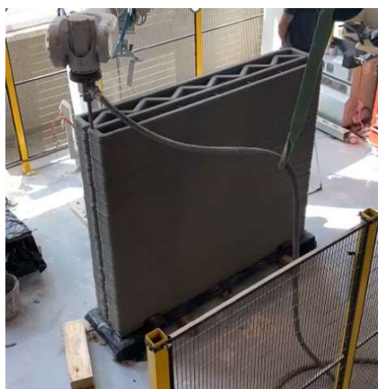
Figure 4-15: Picture of the 3D printed concrete wall during the printing process.
