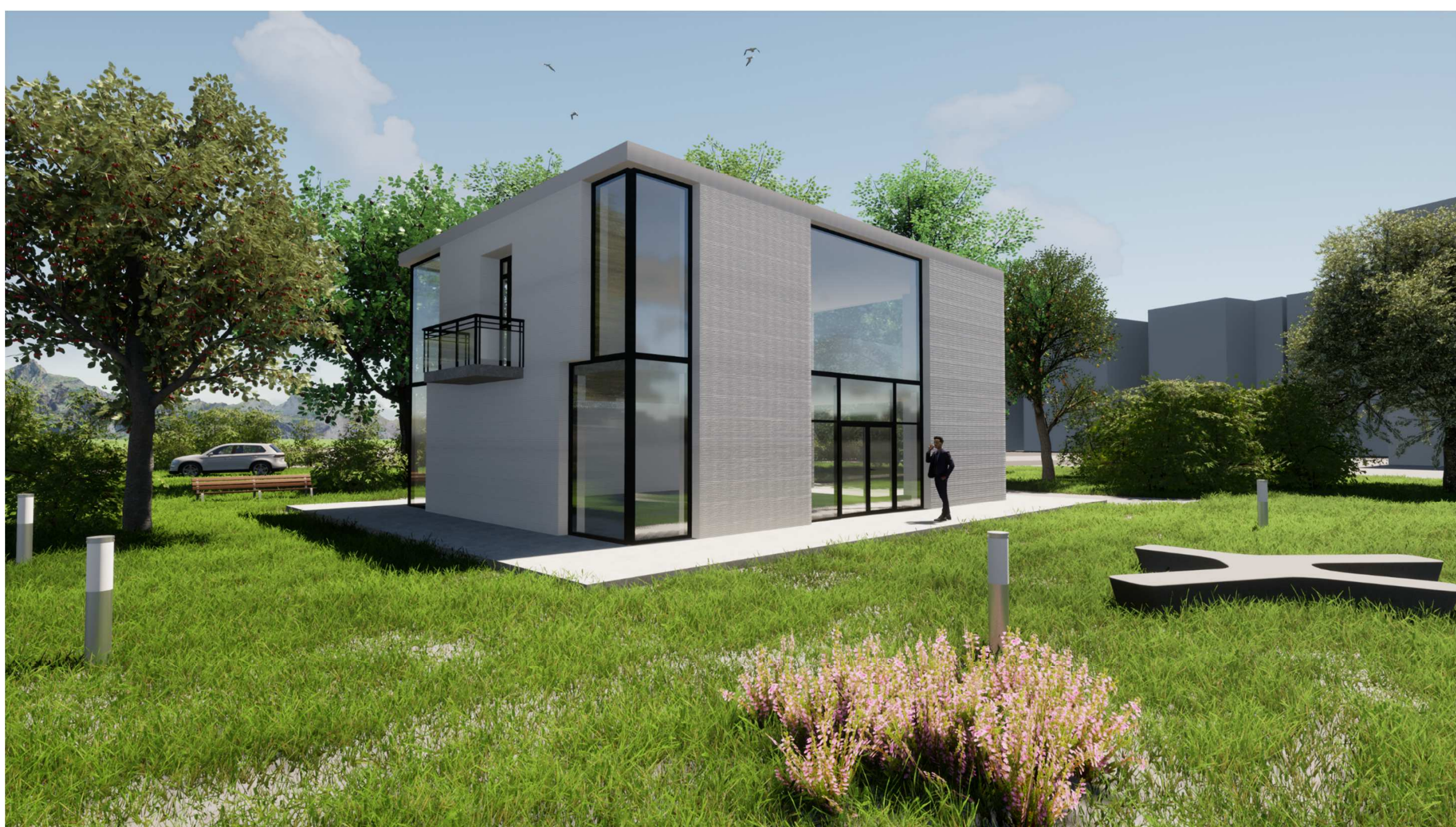
Figure 1. Two storey 3D printed concrete building prototype
