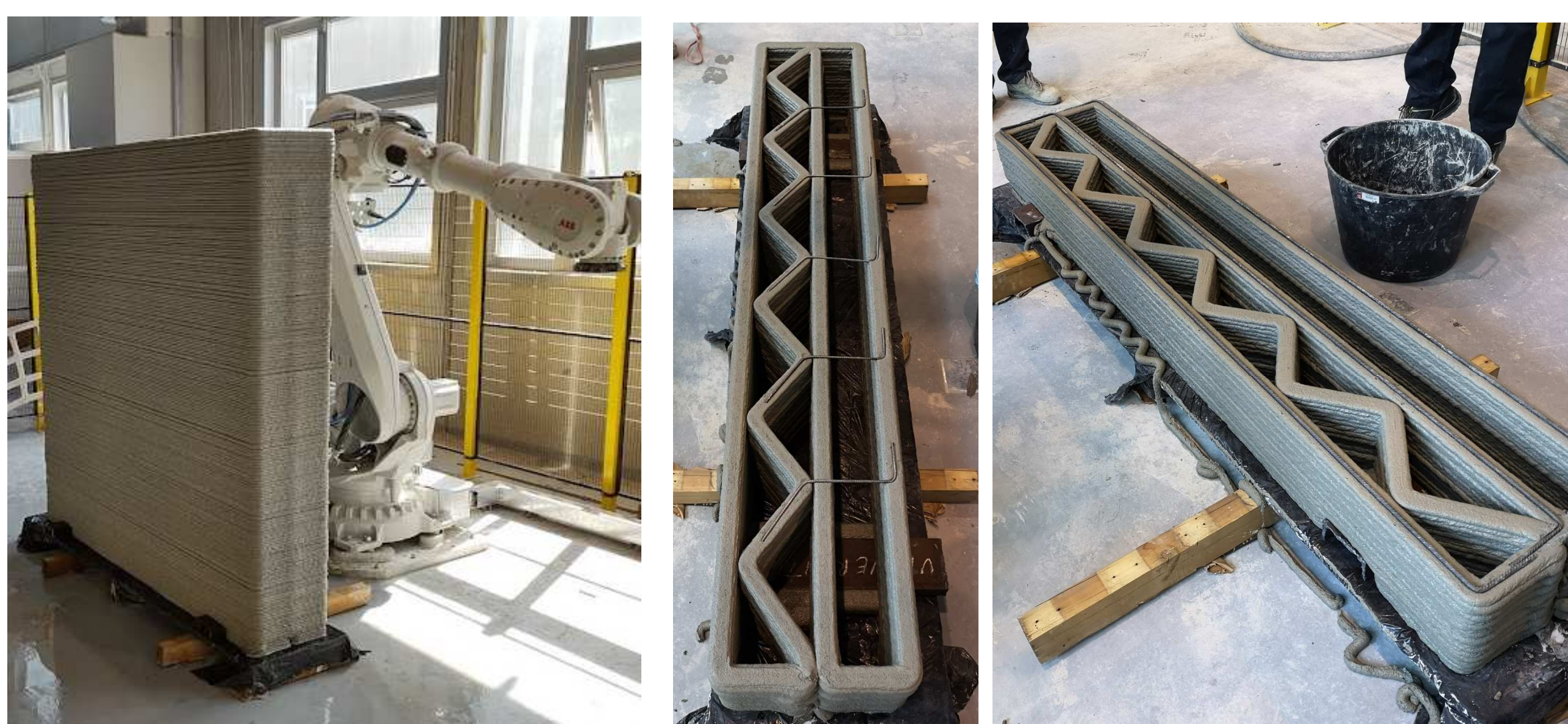
Figure 4. Unreinforced 3DPC wall: printing process.
