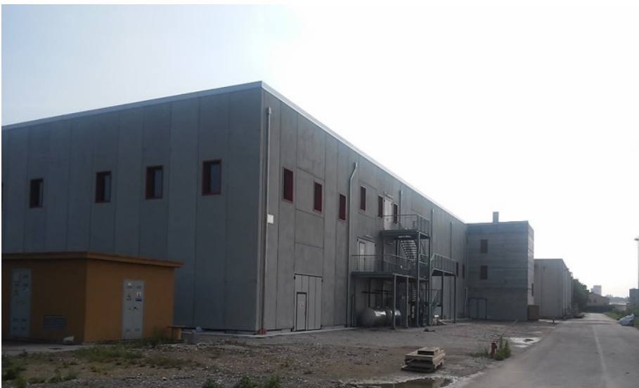
Figure 3.10: The SPES building at LNL.
